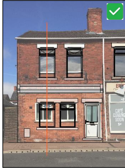
Preferred arrangement. Lower floor windows are aligned with the upper floor and window heads are replicated.
